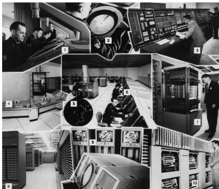
The IBM SAGE Computer Designed, Manufactured, and Installed by IBM for the United States Air Force.
